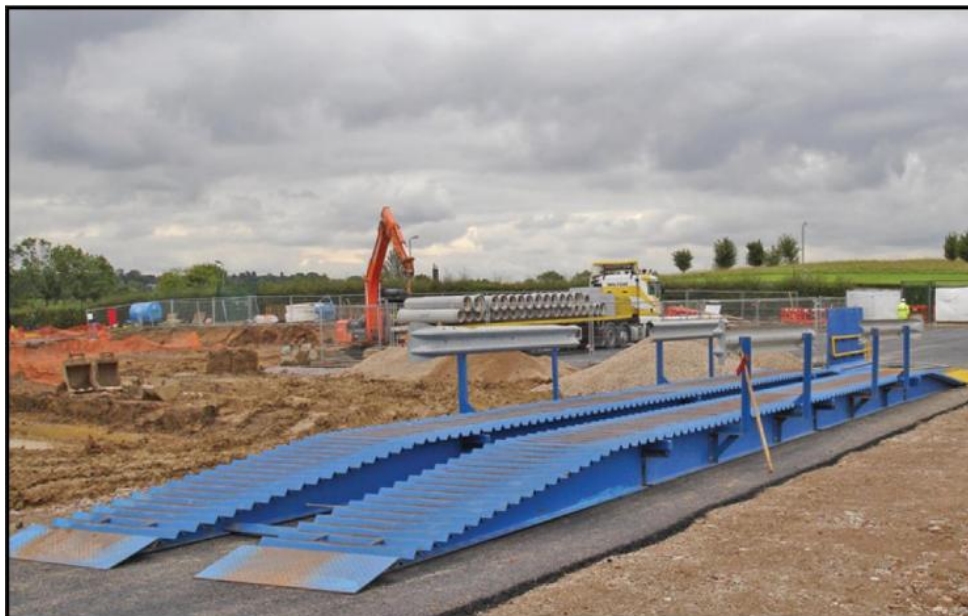
Figure 3-3: Typical Wheel Wash using the Dry Ramp System
